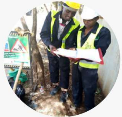
Underground fiber deployment
