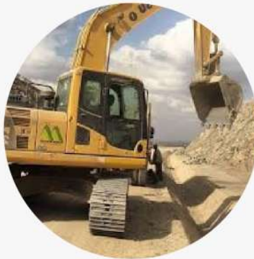
Road Construction Works
